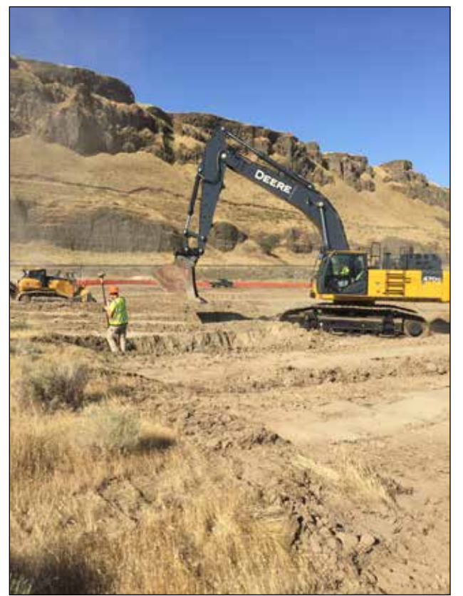
Photo courtesy of Pacific Civil and Infrastructure
