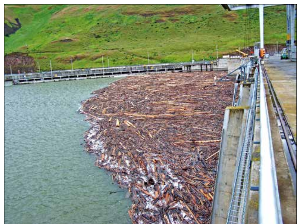
Clockwise from top: (l-r) Matthew Flanagan, Kreg Buryta and Jay Haugen testing the orifice debris plunger. Jay Haugen and Kreg Buryta with their orifice debris plunger device after a successful test on May 5, 2020. Debris built up in the forebay of Little Goose Lock and Dam, 2017.
