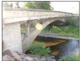
Main Street Bridge
